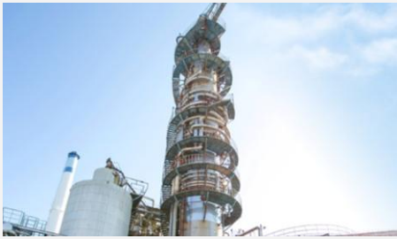
The Kamyr continuous digester used for pulp production
